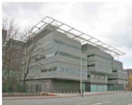
Fig. 1 Alan Turing Building in the university of Manchester.
